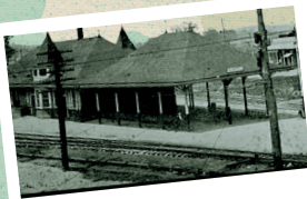
AUSTELL TRAIN DEPOT
